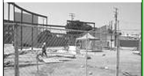
Construction on the new Lindsay Library Branch
